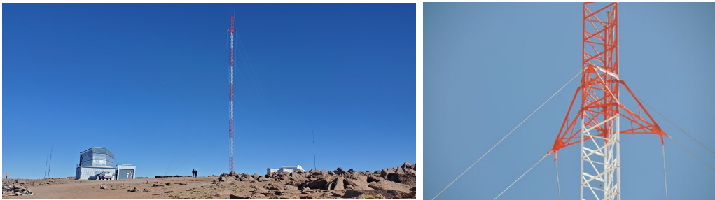
Figure 5.5: (left) Photo of the calibration tower with QUBIC instrument. (right) Photo of the anti-rotational structure, where the calibration box will be placed.
